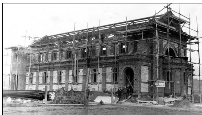
St Theodores Church under construction in 1914
