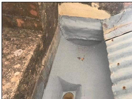
This work was completed in May 2022 and importantly, after experiencing heavy winter rains, there was no evidence of water leaking on to the inside of the sanctuary walls the floors.
